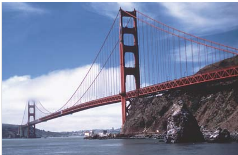
The Golden Gate Bridge is a suspension bridge.
